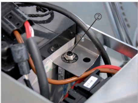
Fig. 113: Secondary safety switch
